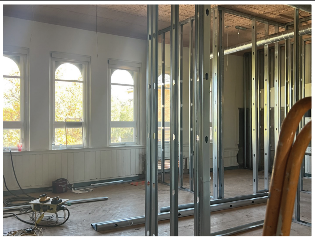
Classroom after asbestos mitigation and with initial framing.
